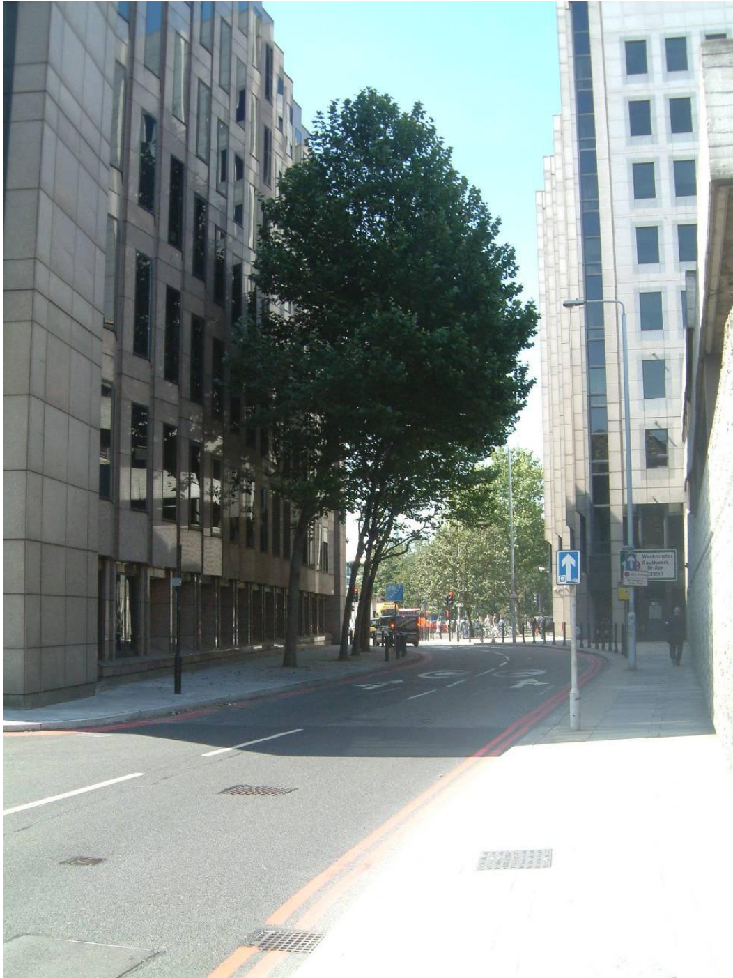
Figure 37: Link C – east to west view
