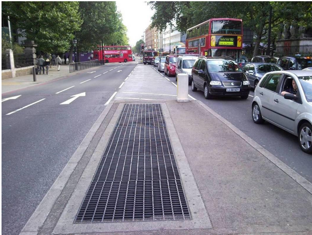
Figure 13: Link A – west to east view
