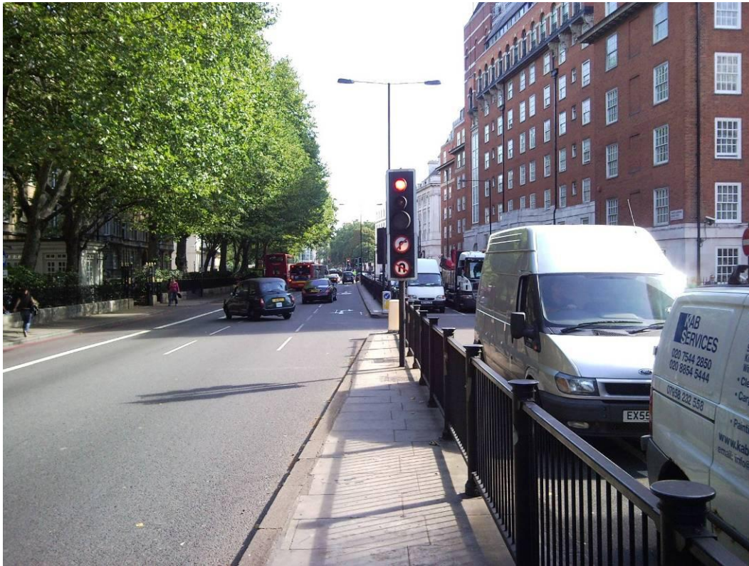
Figure 5: Link C – west to east view
