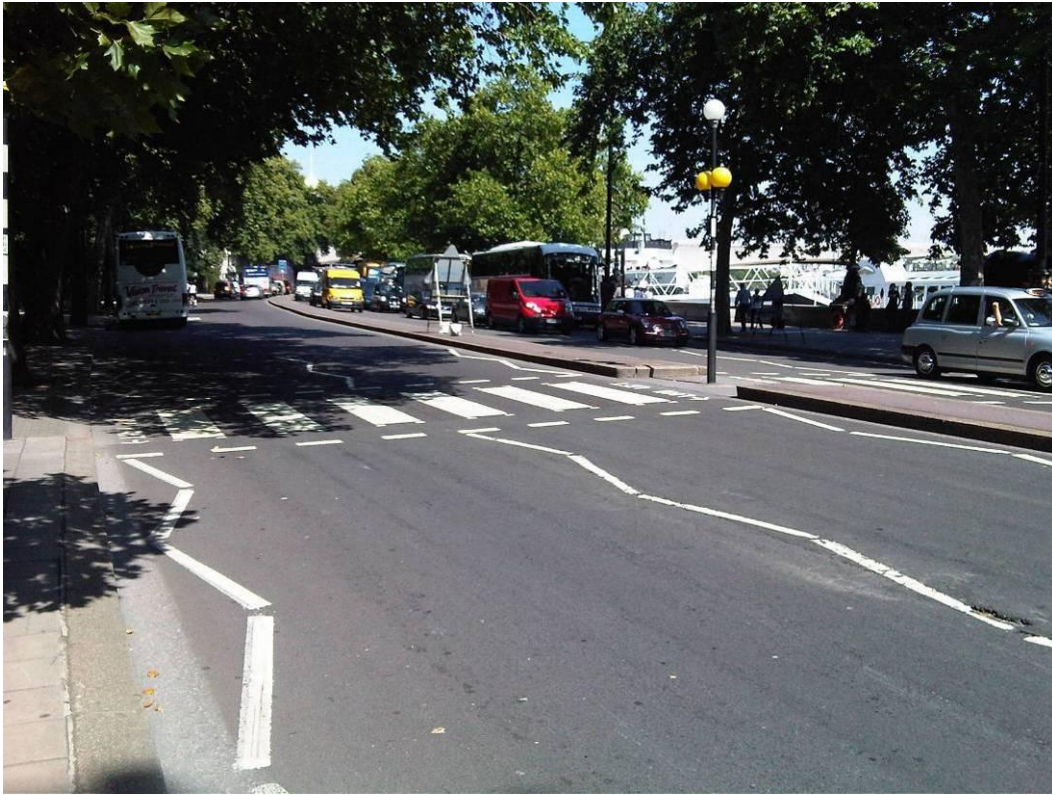
Figure 43: Link C – west to east view
