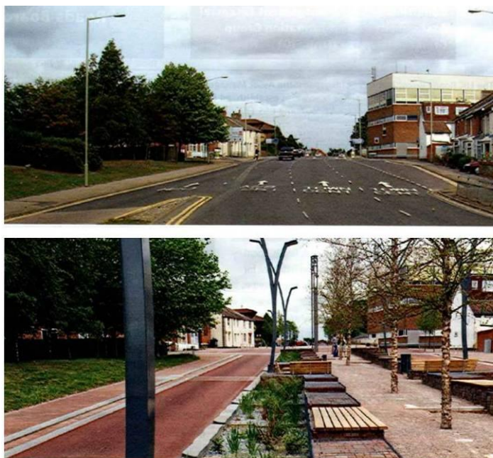
Figure 4: Ashford ring road before and after reconstruction 19 .
